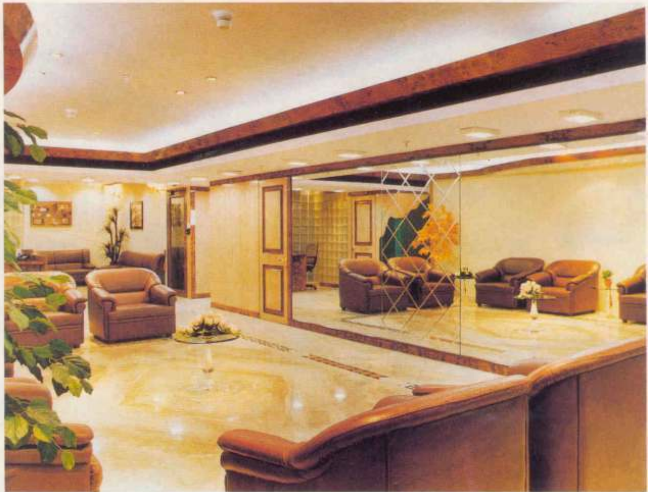
Second floor lounge : Indirect lighting, smoke alarms and sprinklers can be seen on the ceiling . The sides above the A/C grills have veneer finish. Mirrored walls add to the visual space. Flooring is Italian marble
